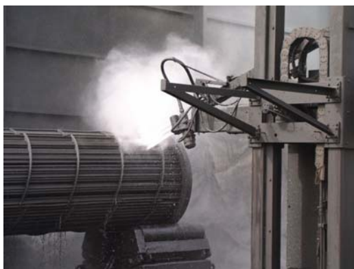
Fig.: External cleaning of crude oil exchangers
